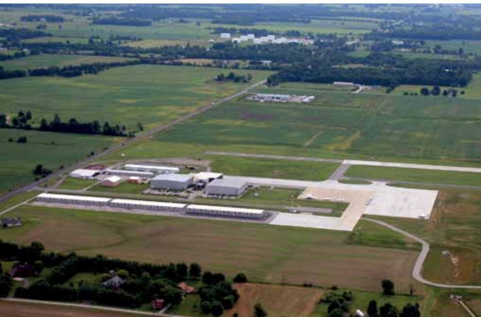
Aerial showing expanded parking ramp south (right in image) of the terminal.
