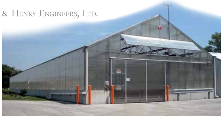
BioSolids Solar Drying System at the Wastewater Treatment Plant
