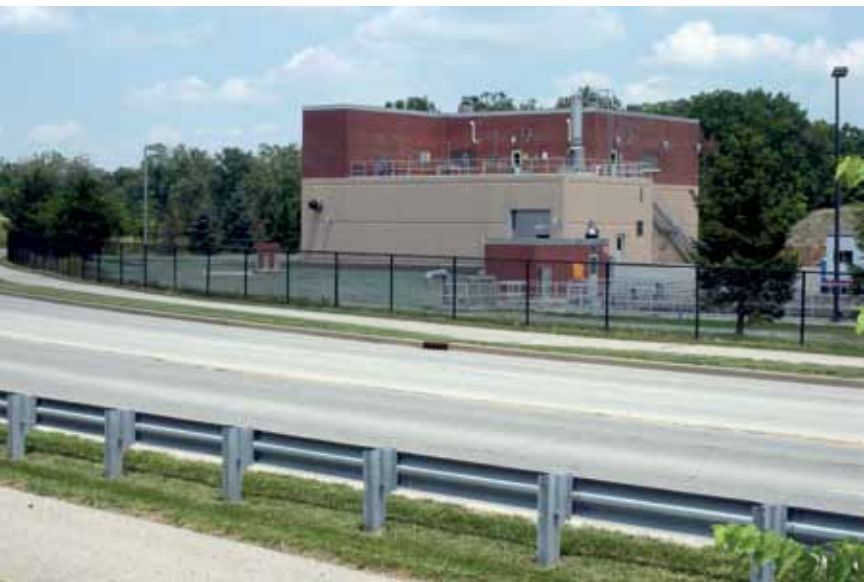
Headworks Facility at the Wastewater Treatment Plant
