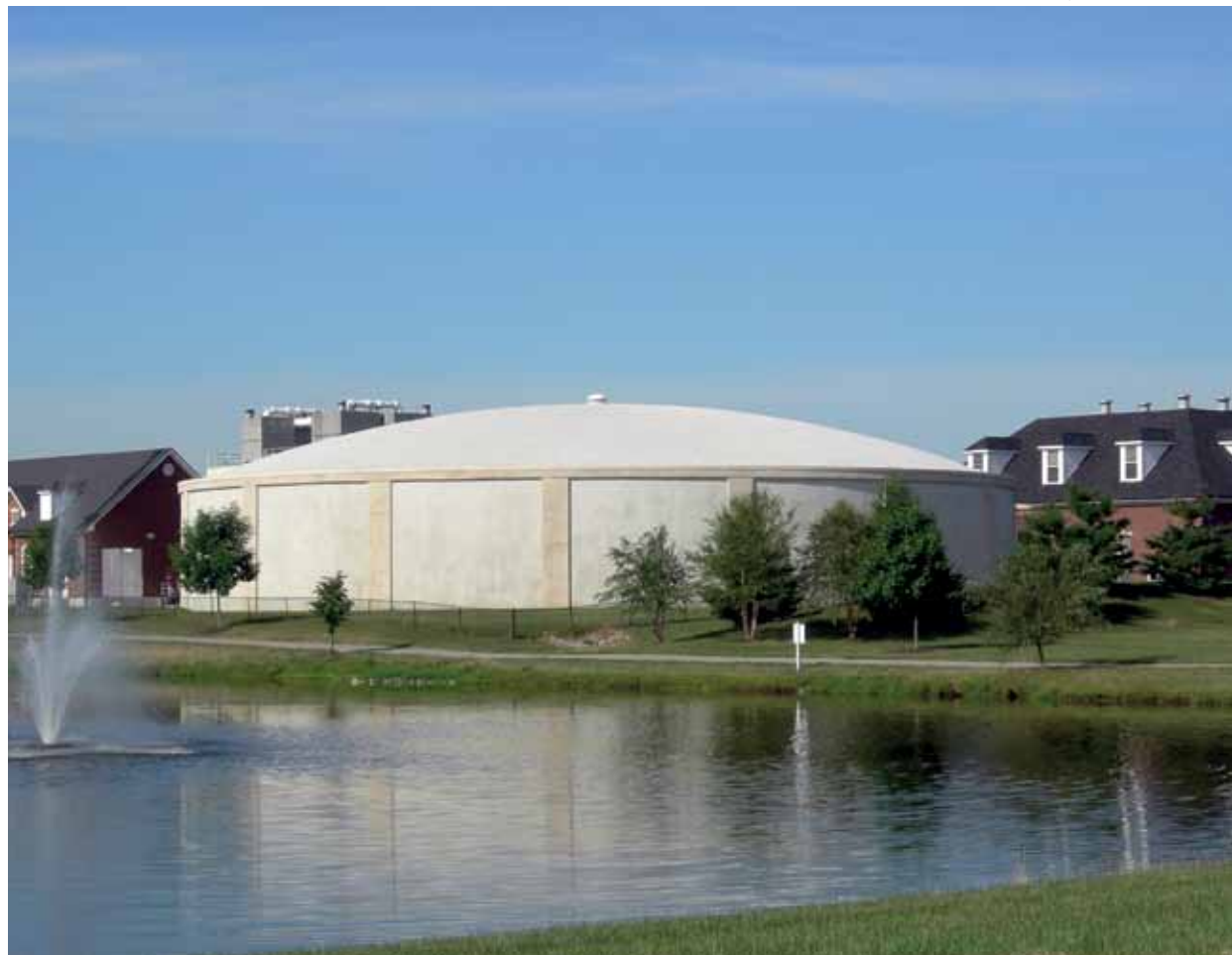
Finished Water Storage Tank
