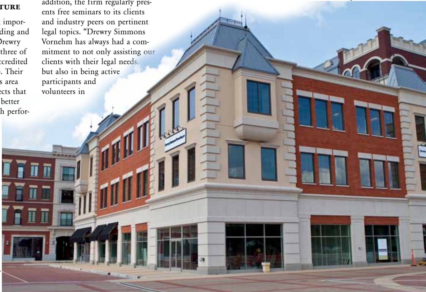
DSV's Carmel City Center office.
