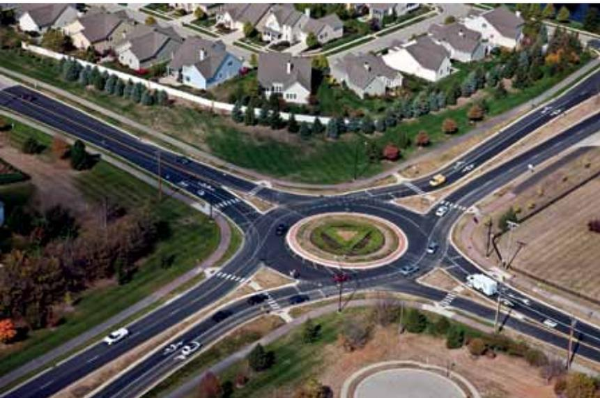
allow for freer vehicular flow, reduce vehicular accidents, eliminate the need for traffic signals, and improve travel time. Since 1996, American Structurepoint has helped develop more than 100 roundabouts. The City of Carmel, now dubbed "Roundabout City," boasts over 80 roundabouts either in place or under construction
